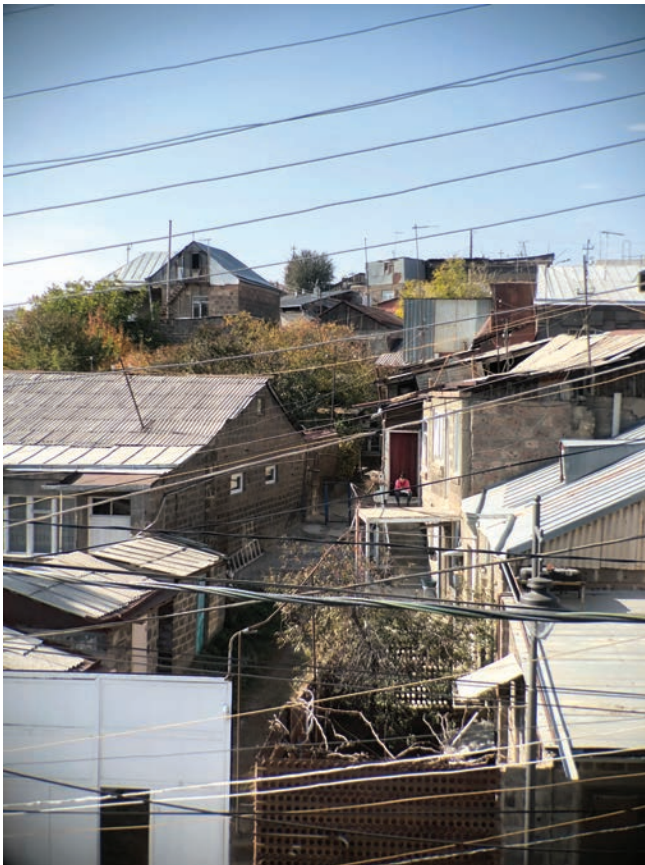
Gyumri Electric Lines 2019. Photo: Suzi Banks Baum.
